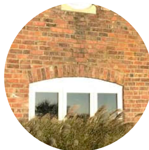
Arched brickwork
